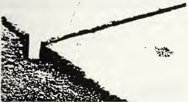
Fig. 3.2.2.1 — Faulting (stepping)
